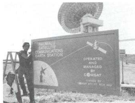
Visitors to the Paumalu Earth Station are now greeted by a new sign painted COMSAT blue with white lettering at the station's main entrance. Seen erecting the sign are Bill Romerhaus and Jeff Doran of the Facilities crew.
