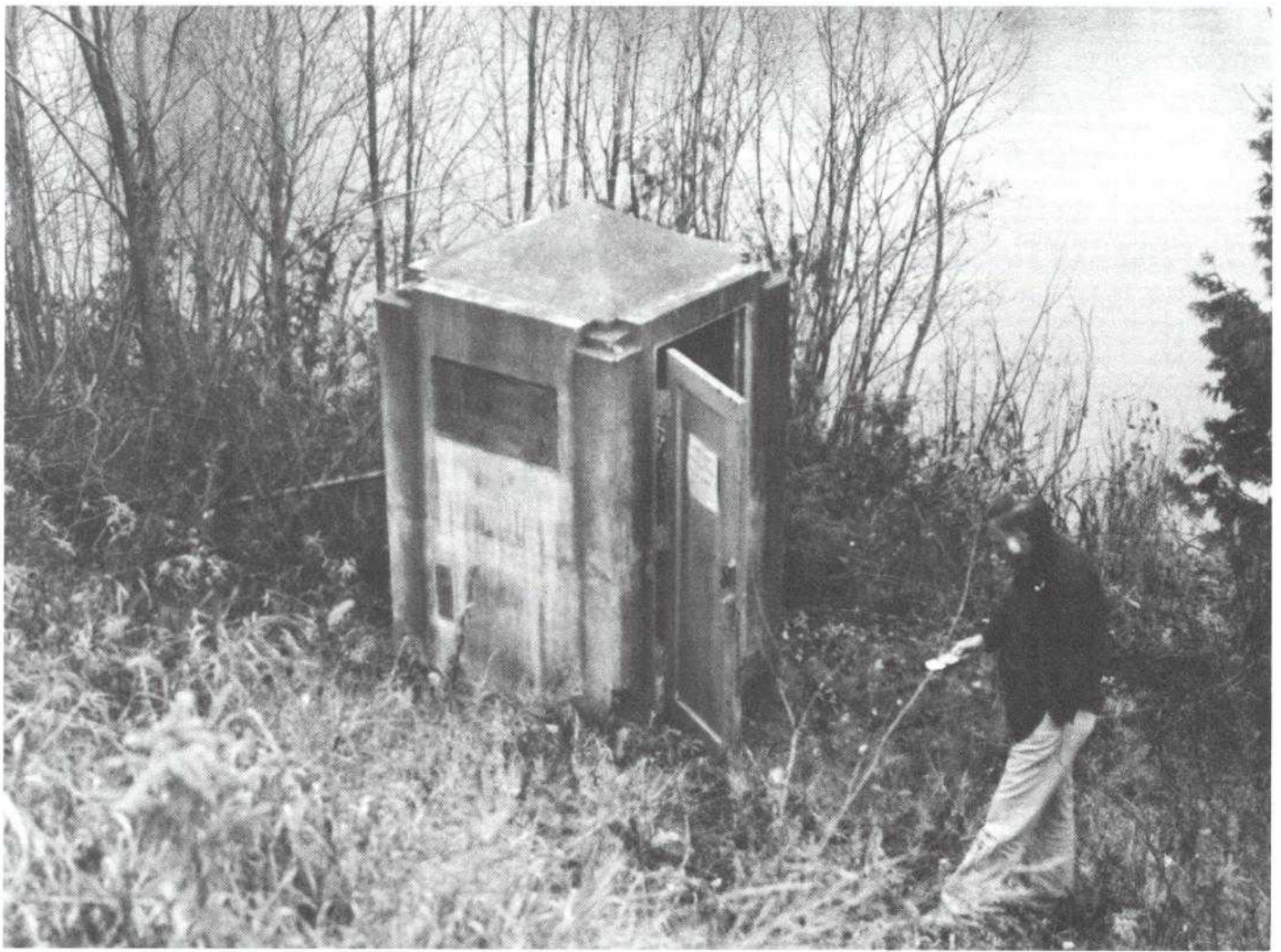
A protective shelter for water-height recording equipment by the Meduxnekeag River near Houlton, Maine. Gus S. Souris, Jr., of COMSAT General checks shelter position with a compass.
