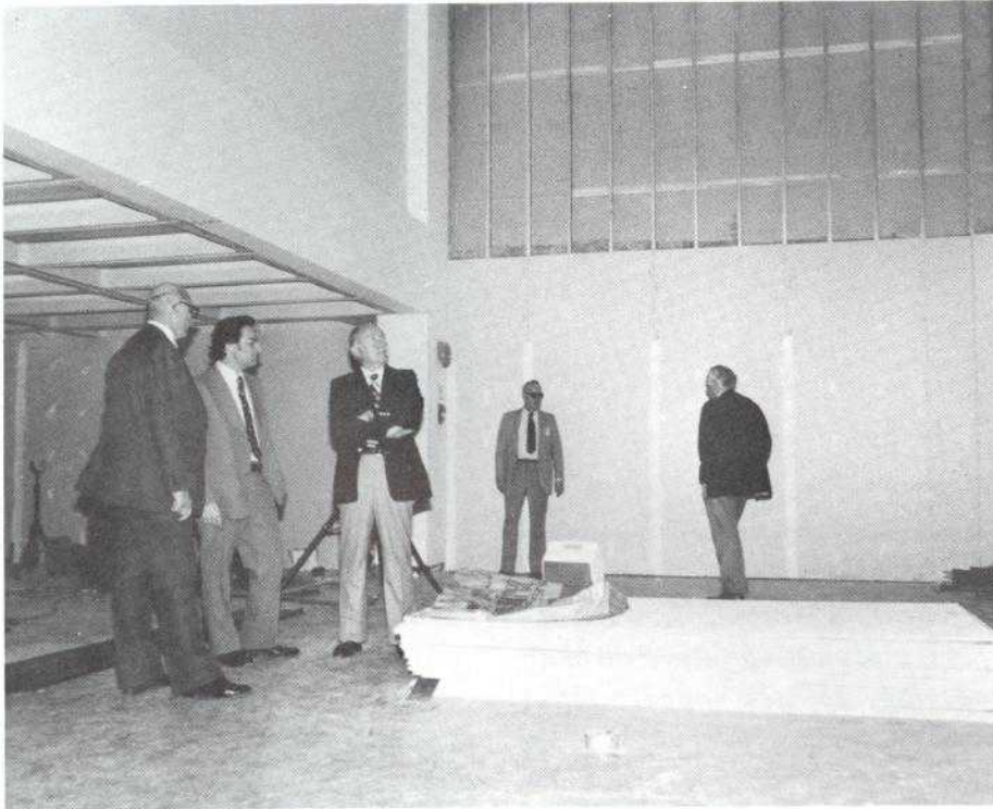
The new Launch Control Center, which is a project of EIG's Control Systems Engineering Division, is shown during an early stage of its construction on the ground floor of the L'Enfant Plaza headquarters building. The three men in the left foreground are, from the left, Gene E. Christensen, Manager, Facilities and Office Services; Brian J. Williams, Director of EIG's Control Systems Engineering Division; and Edward J. Sanderson, Director, General Services. The two men in the rear are outside contractors.
