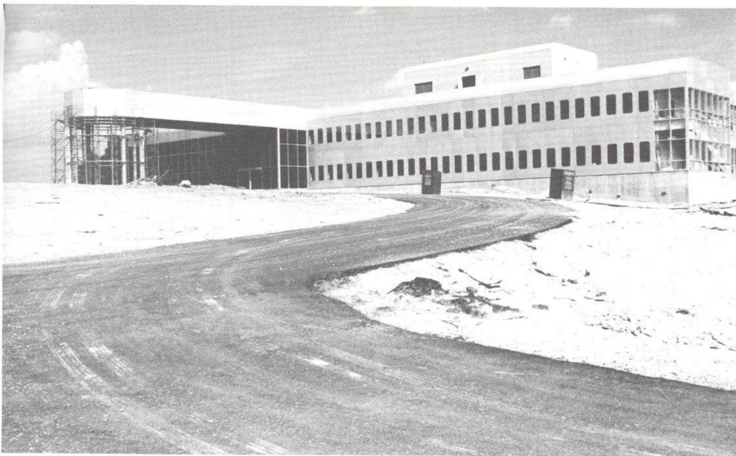
Construction is nearing completion on the new COMSAT Labs at Clarksburg, Md.
