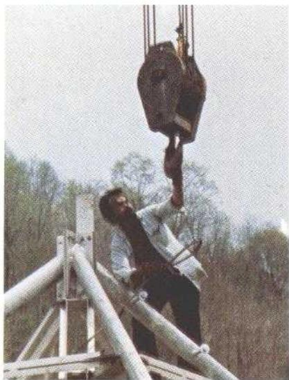
*Once dish was in place, the quadripod structure was lifted from the ground and set inside it. Here a worker prepares to attach crane hook to the top of quadripod.*
