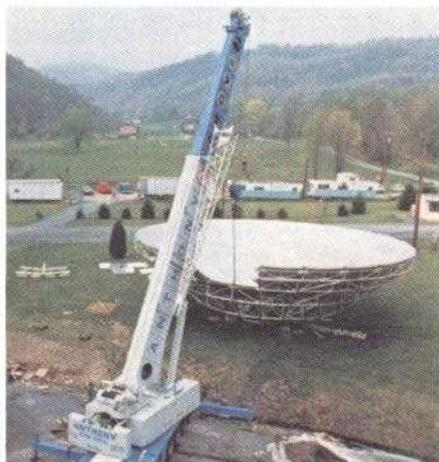
*The 62-foot diameter dish rests on an area of lawn where it was constructed. A short time later, the 120-ton crane began the lift.*
